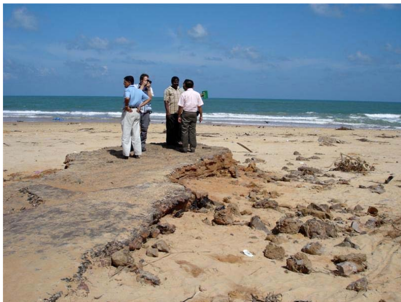
The devastated coastline of Mullativu, 3 days after Tsunami struck. The entire section of the main road here has been washed out to sea. (Photo by Kolitha)
